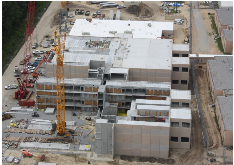
Above: Since last November two large cranes have been stacking the new precast inmate cells into place.
